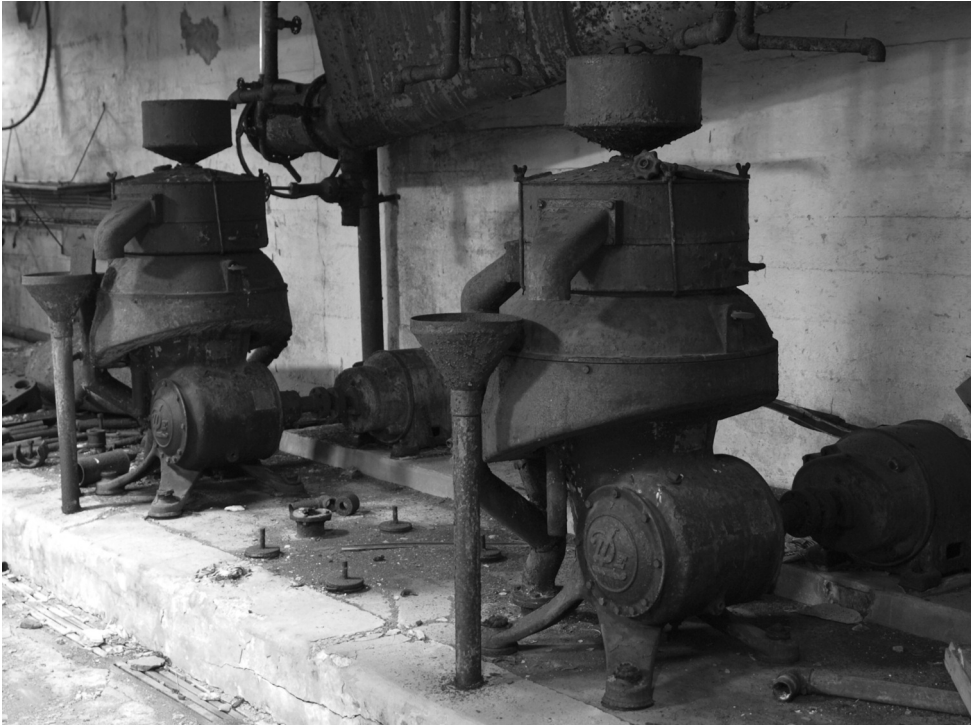
Figure 1.10 Releasement. Centrifugal separators in the herring factory at Eyri Photo: Bjørnar Olsen
