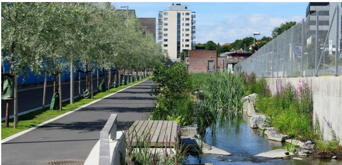
Figure 4. Hovinbekken at Hasle. Photo: Agency for Planning and Building Services.
