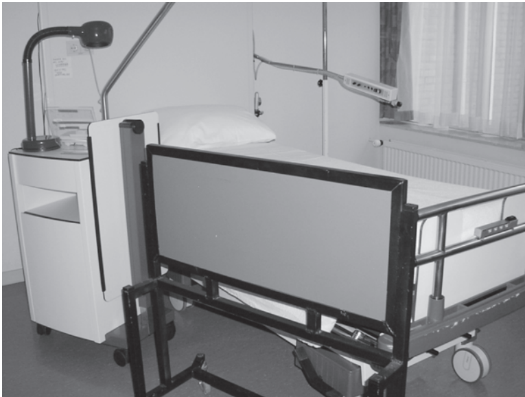
Figure 4.9 A lead screen close to the bed in a brachytherapy room, to be used for patients who need more intensive nursing care. The screen contains 2 cm Pb thickness.
