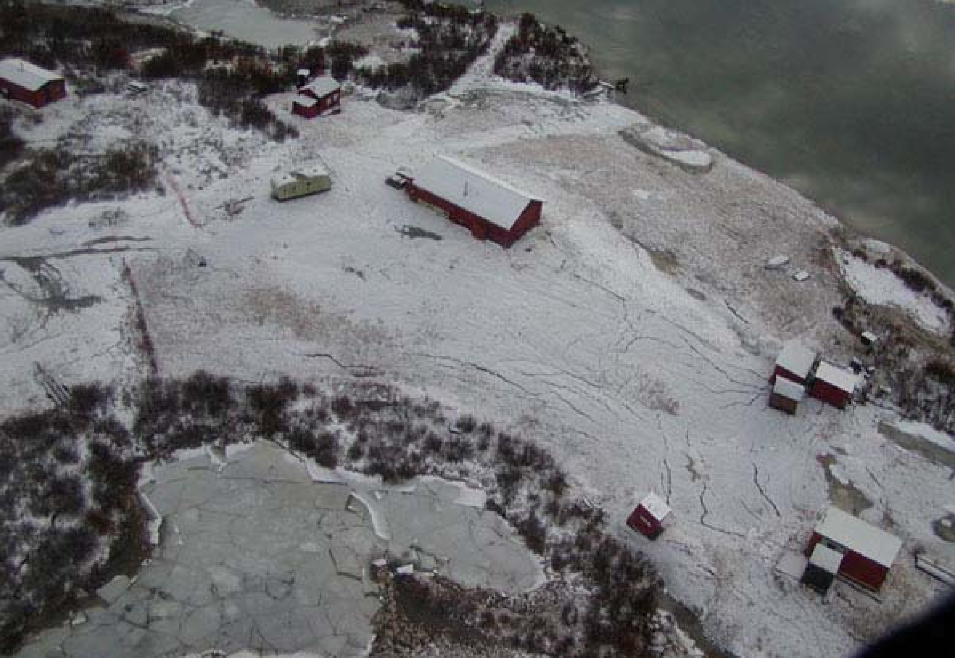
Alaska earthquake 20021102 liquefaction at Fielding Lake
