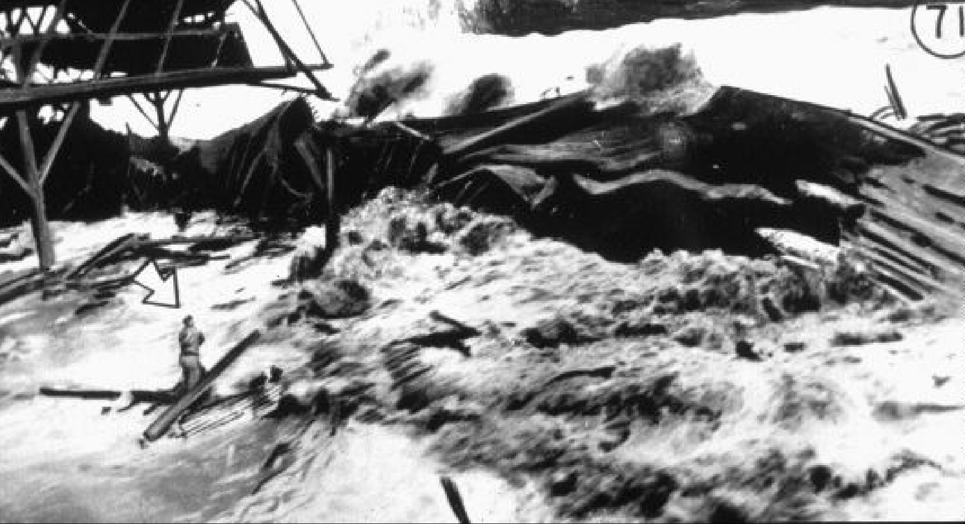
Tsunami breaking over Pier No. 1 in Hilo Harbor, Hawaii, 1975.
