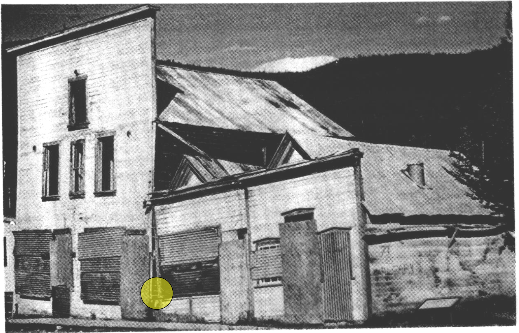
Plate II: Building Showing the Results of Thaw Settlement in Dawson City, Yukon Territory, Canada.
