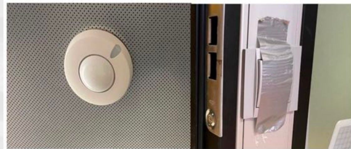
Fig. 2. Left: Motion sensor mounted in the ceiling of the offices. Right: Button disabled with gaffe tape.
