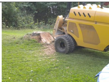
Figure 7: Stump grubber removing the tree stump.
