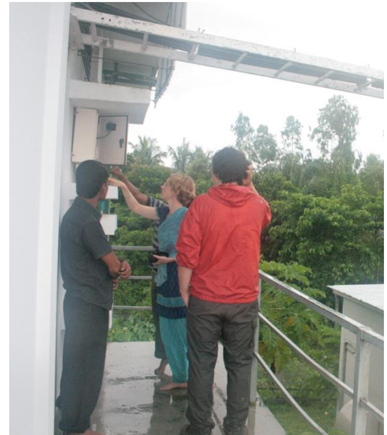
Moving the main circuit breaker to the outer wall
