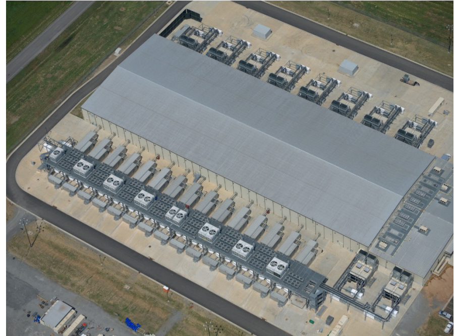
Google Data Centre at Mayes County, Oklahoma
