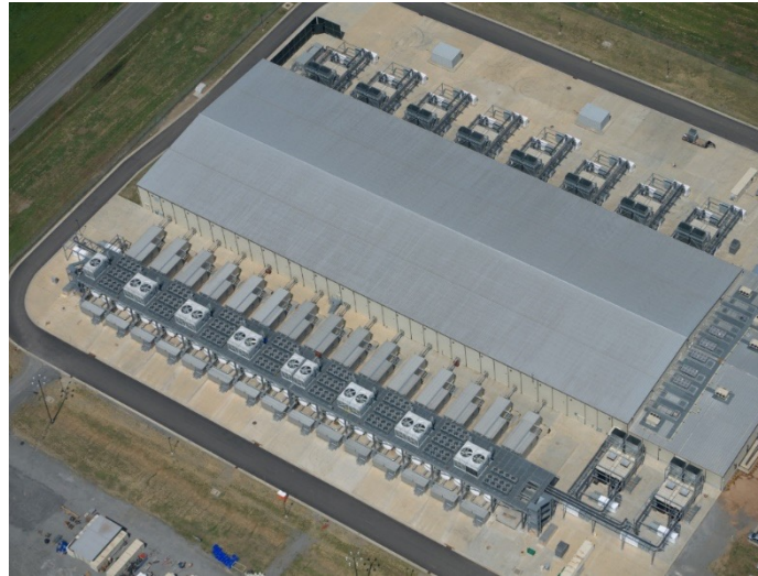
Google Data Centre at Mayes County, Oklahoma
