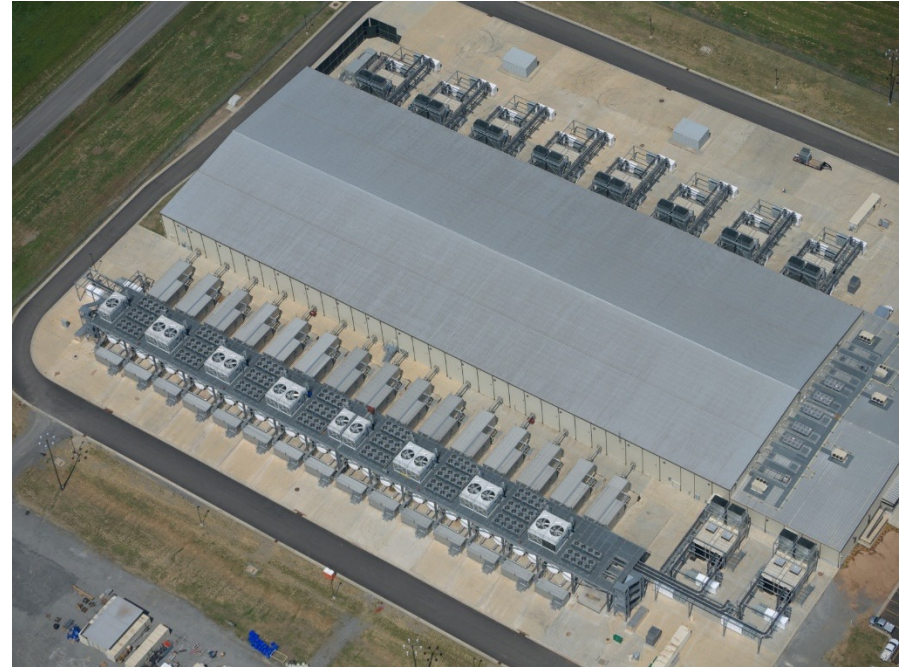
Google Data Centre at Mayes County, Oklahoma
