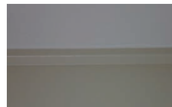
Overgang vegg/himling m/taklist
